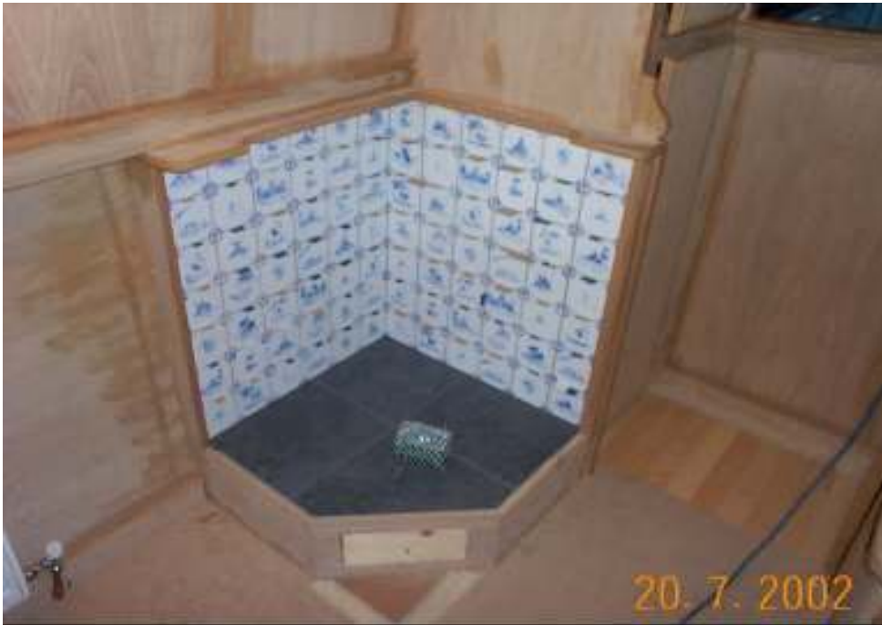
DELPH TILED FIREPLACE UNDER CONSTRUCTION.
