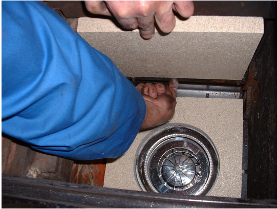
Fit the second front board
