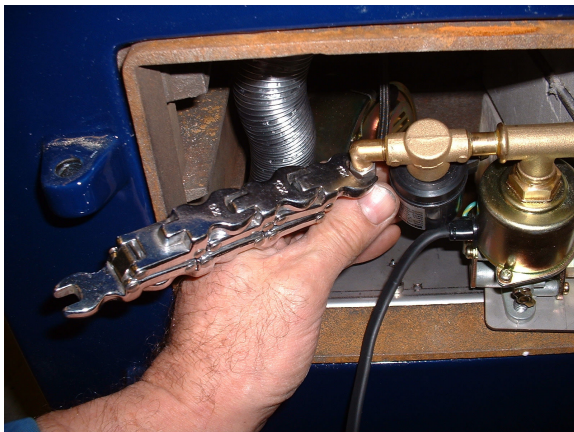
Fig 21 Tighten the fuel hose.
