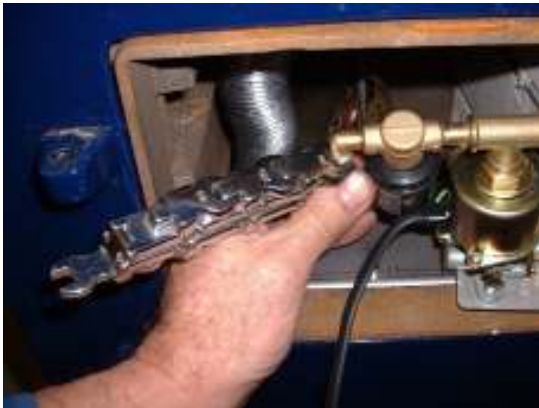
Fig 21 Tighten the fuel hose.
