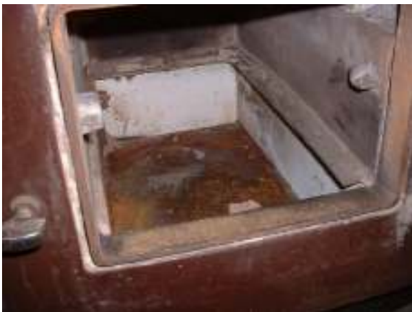
Fig 13. Remove the ash pit base plate casting.
