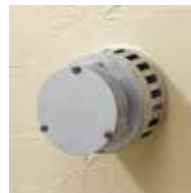
Balanced Flue (No chimney required)
