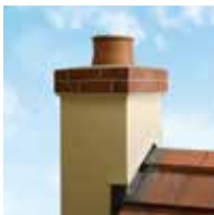
Brick or Stone Chimney (Class 1)
