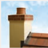
Brick or Stone Chimney (Class 1)
